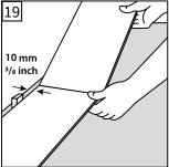
Mark the required length of the last floor-board of each row. For this purpose, use a square or, if not exactly perpendicular to the wall, a sliding level. Then score the element with the installer's knife, two or three times on the decor side along the marking. At that point, break the element over a straight edge (table edge or the like) and pull the two parts apart downwards at the resulting predetermined breaking point (decor side facing upwards).
